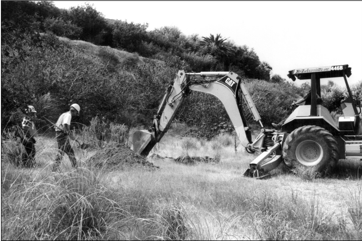
Figure 27. Trenching at LAN-62.
