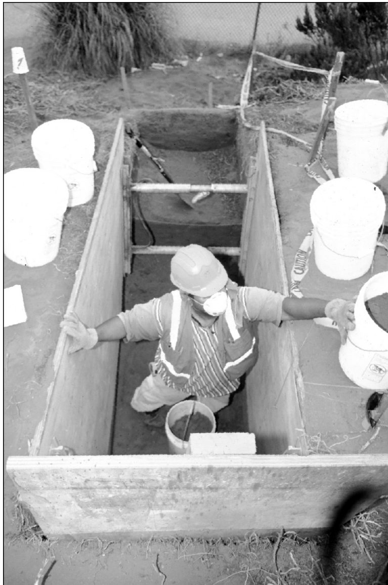
Figure 32. Shoring in units at LAN-211/H.
