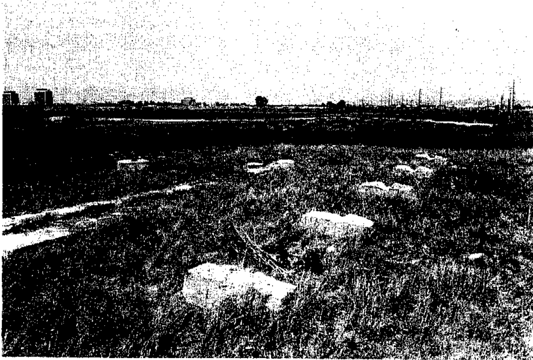
Figure 55. Feature 1, a Series of Concrete Block Supports for a Pipeline at SR2, Facing North.
