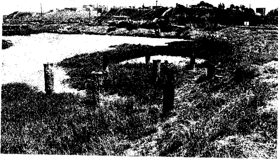
Figure 58. Feature 6, Wooden Pier Remnant at SR2, Facing Southeast Toward the Ballona Escarpment.
