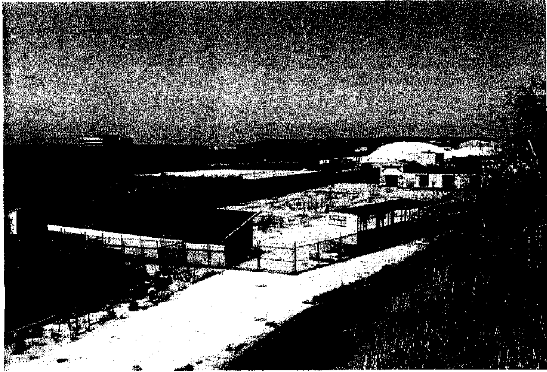
Figure 78. West Portion of SR 17, the Howard Hughes Industrial Complex within Area D, Facing North.
